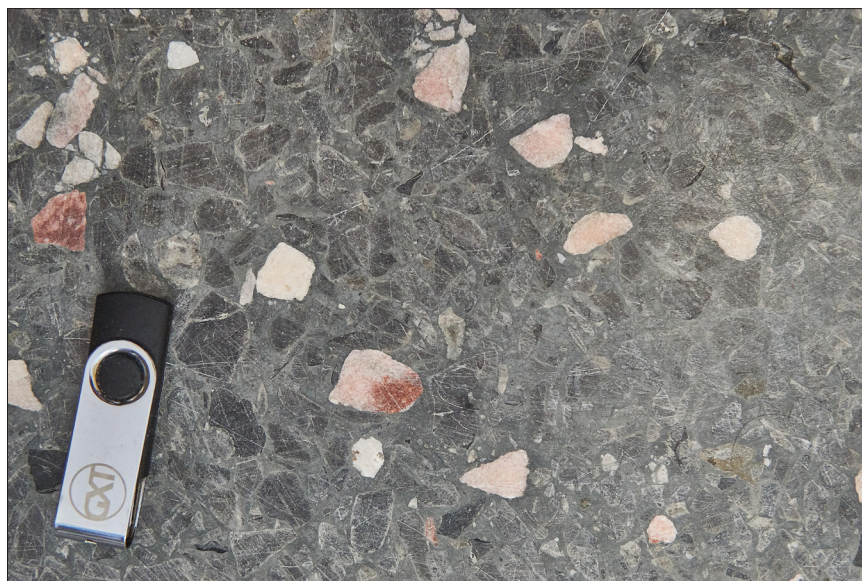
Figure 2. Typical terrazzo tile from the hallways of Sciences de la Terre, Université du Québec à Chicoutimi, with USB stick as scale; see also Figure 3.
